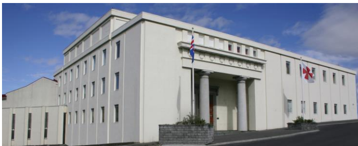
The Masonic Hall in Reykjavík.
