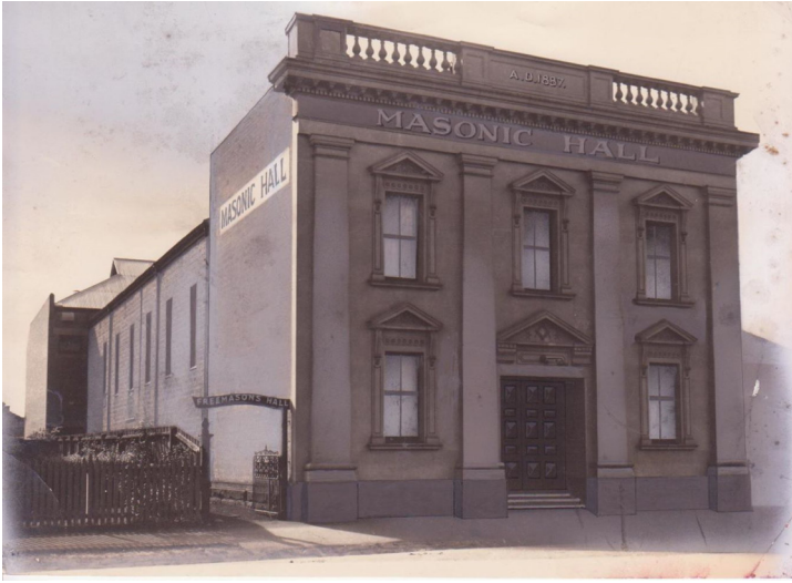
Fig. 2. Ascot Vale Masonic Hall. Photo used with kind permission from Gordon Lodge No. 99. Taken from Gordon Lodge: An Historical Sketch on the Occasion of the Jubilee Celebrations (Private publication, 1986), 20.
